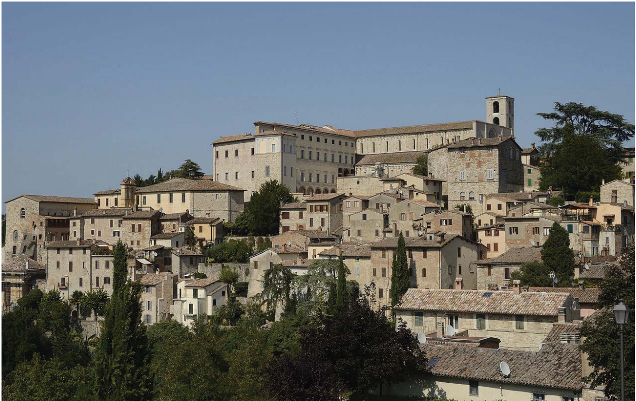
Todi (above) and its walls (below)
