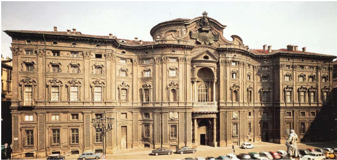
Façade of Canigiano-Guarini Palace
