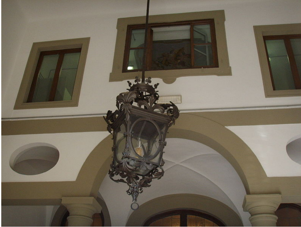
Entrance of the Nunziata Guadagni Palace –detail (crown of marchese on top of the lamp)
