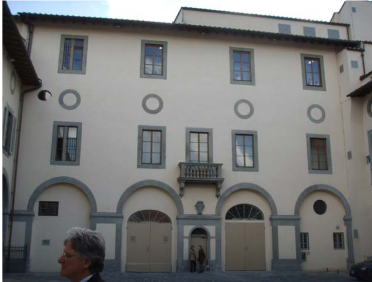
The stables on the ground floor. You can see the size of the Guadagni Palace by the size of the two women under the family crest.
