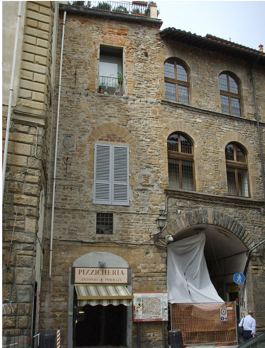
Middle-Ages houses in De' Pazzi Corner. These were probably owned by the Guadagni in the Middle-Ages.
