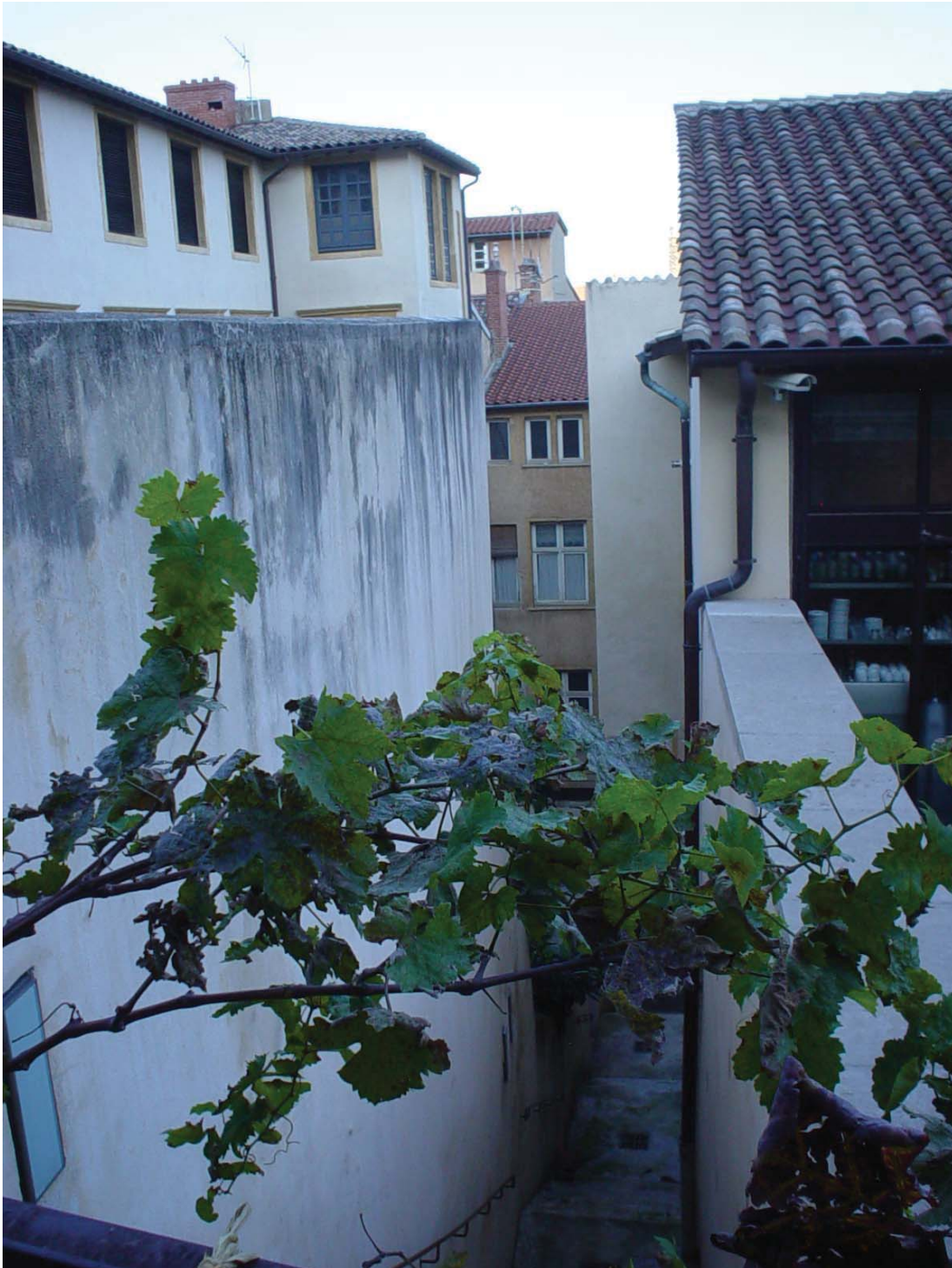
NARROW STEEP STAIRCASE LEADING FROM THE "GRASSY BACKYARD" TOP OF THE MUSEUM DOWN TO GUADAGNI STREET. ALL THE BUILDINGS IN THE PICTURE BELONG TO THE MUSEUM. THE IMMENSE GUADAGNI PALACE USED TO INCLUDE A LARGE PART OF LYON. LET US REMEMBER THAT IN THE 16TH CENTURY THE GUADAGNI WERE NOT ONLY THE RICHEST FAMILY OF LYON AND OF FRANCE, BUT ALSO OF ALL OF EUROPE.
